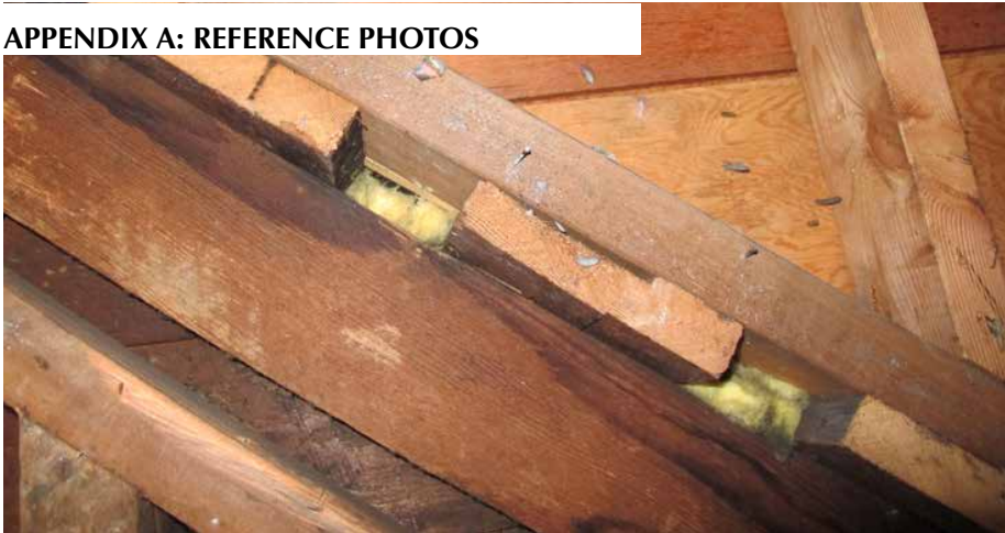
Cut-through roof structure showing original nailing strips.
