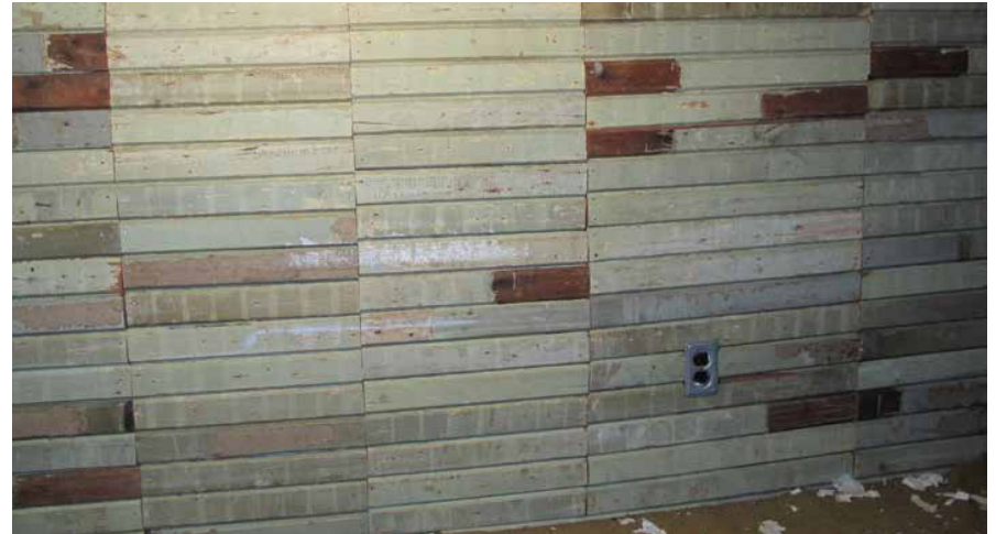
Basement Level wood sidings repurposed as cladding
