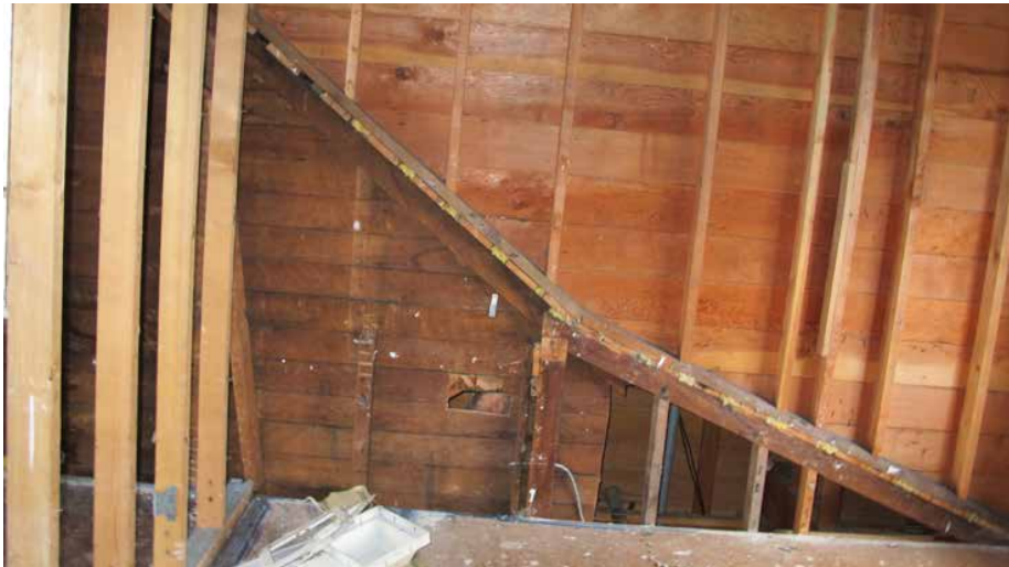
Siding behind later construction, Ground Floor East Side
