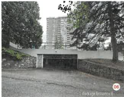
Parkage Entrance B
