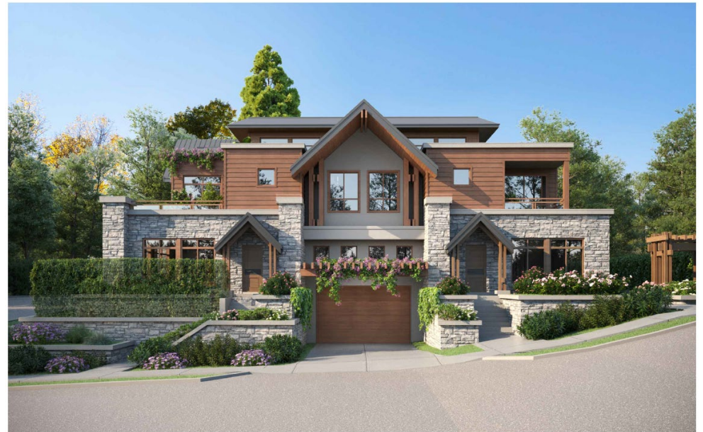
VIEW FROM 29TH STREET
