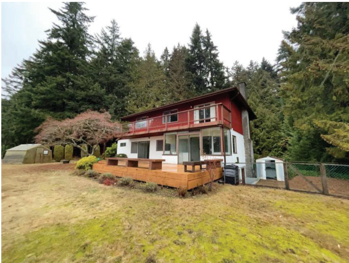
Photo 1. View of the house currently on site, looking north.
