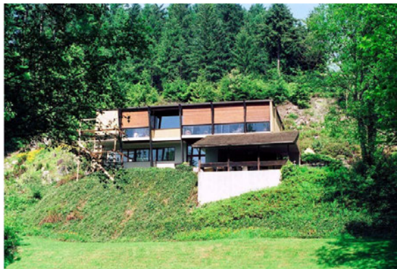
Figure 1: Photo of the Lauder Residence
