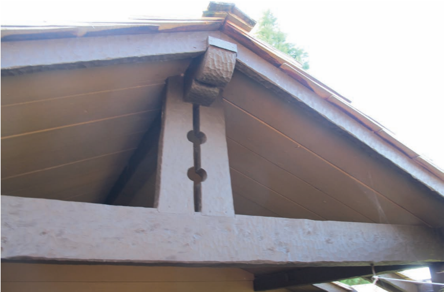
Gable end detailing on roof above rear patio
