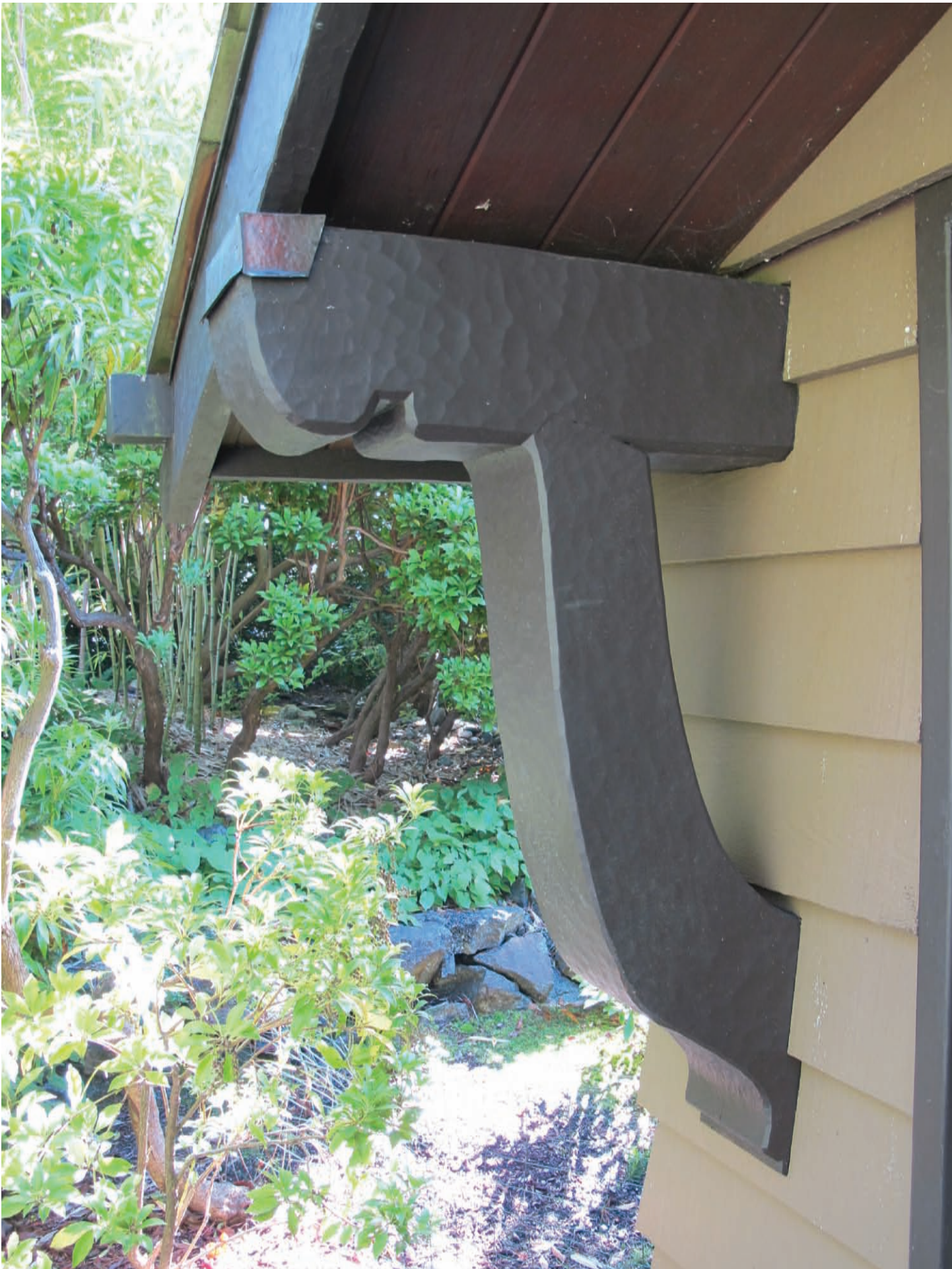
Hand adzed curved wooden bracket
