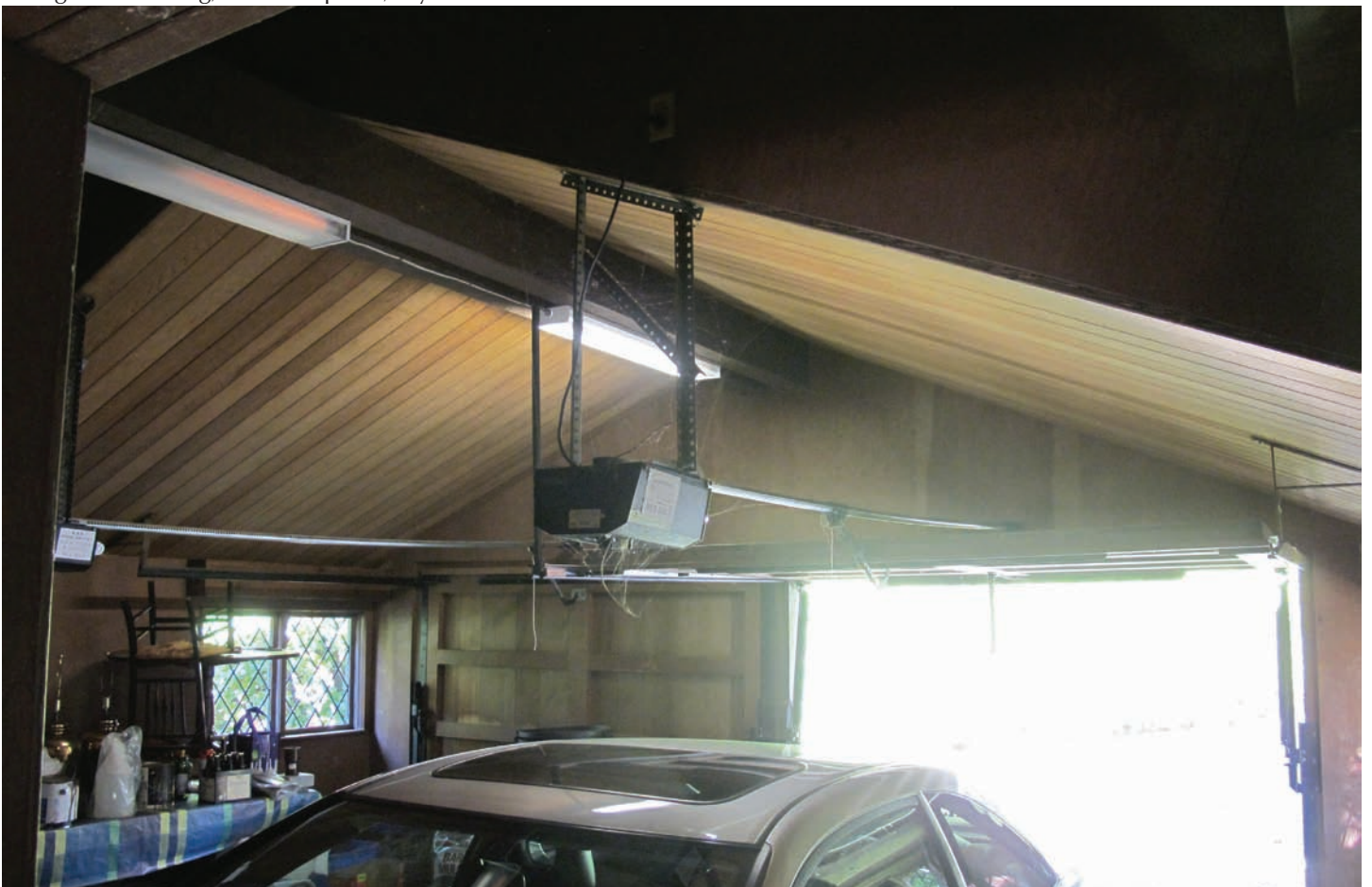
Vaulted garage ceiling
