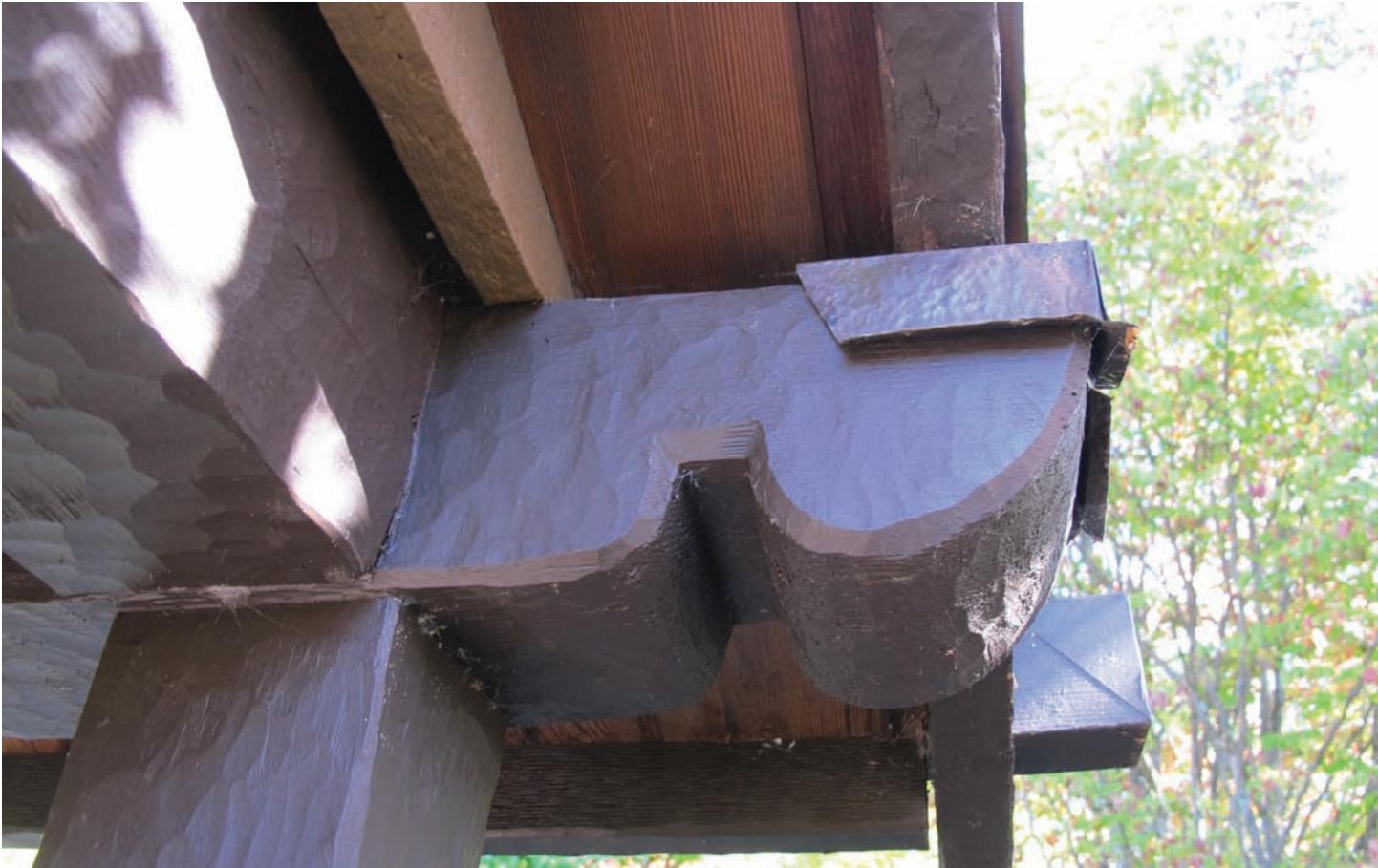
Hand adzed wooden bracket
