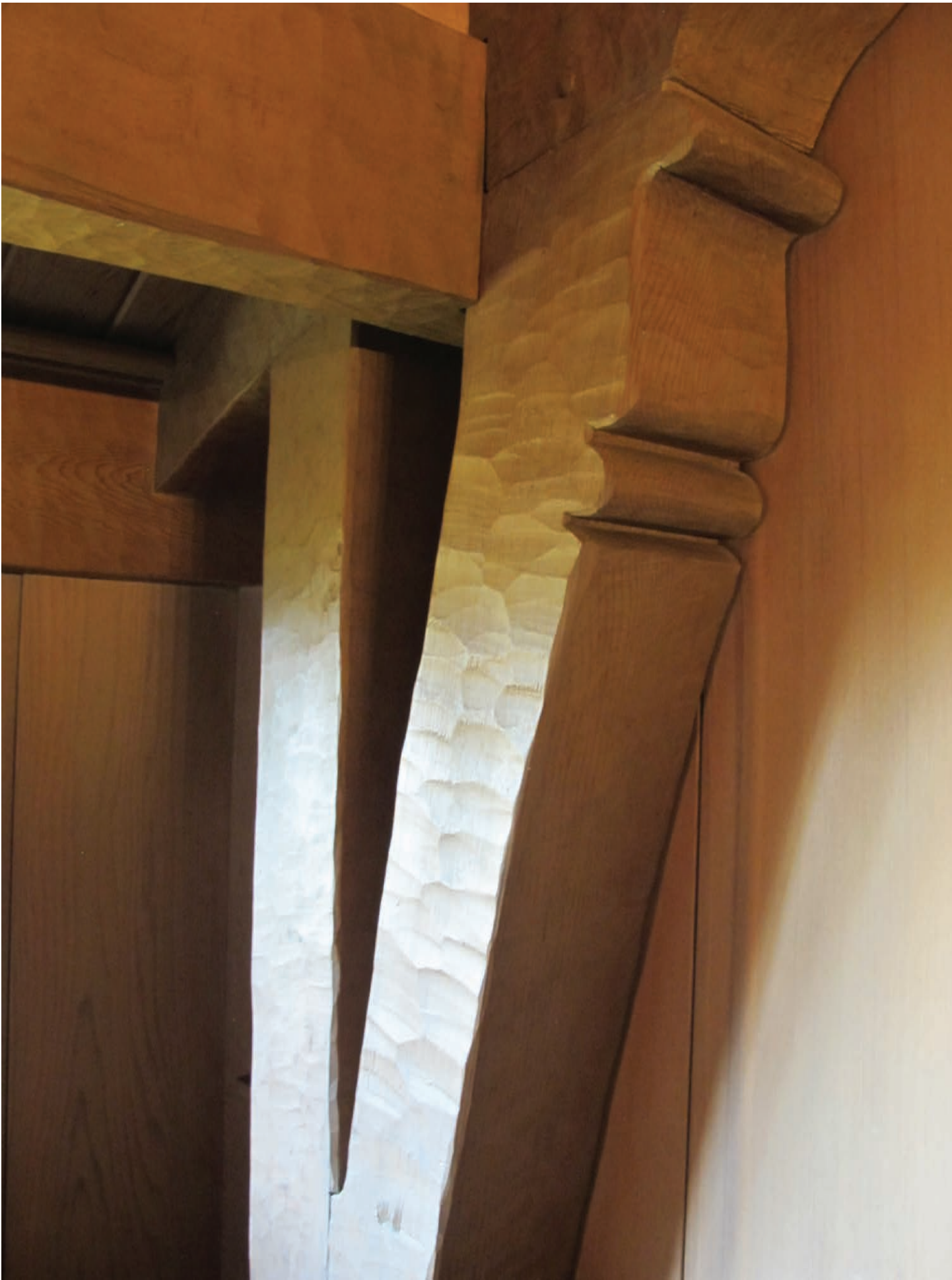
Hand adzed wooden scroll cut post
