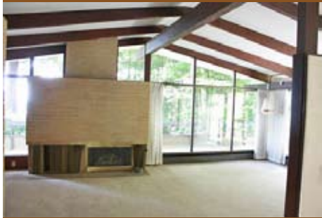
Above & Below: Living room facing south with brick chimney and fireplace
