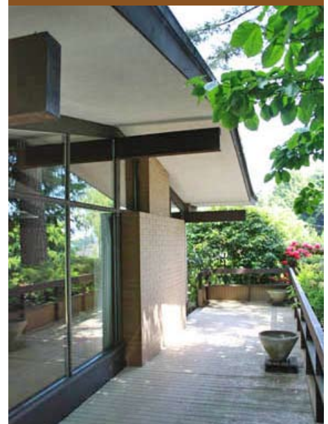
Cantilevered 2nd floor carport
