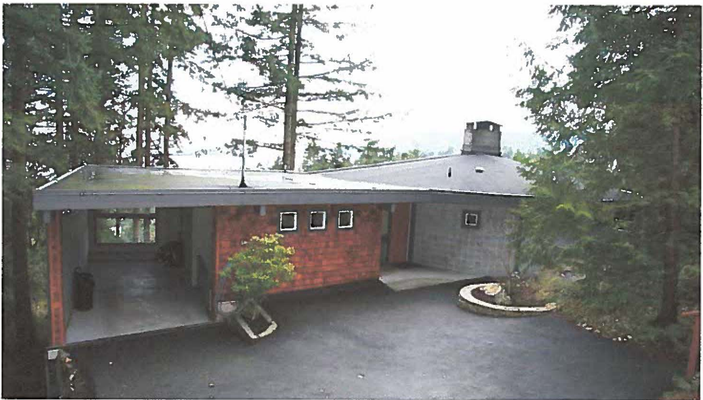
Front facade with open carport and curved library wall
