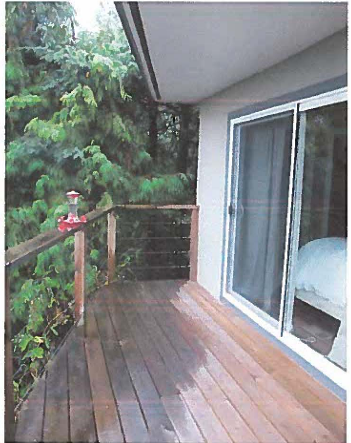
New south deck and new sliding doors
