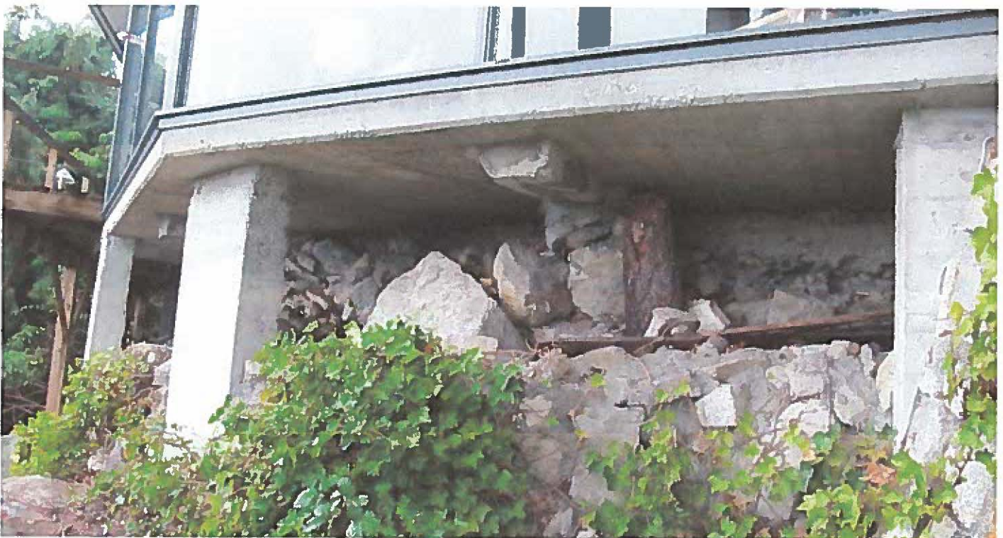
Concrete pillars support the cantilevered floor slab of the living room
