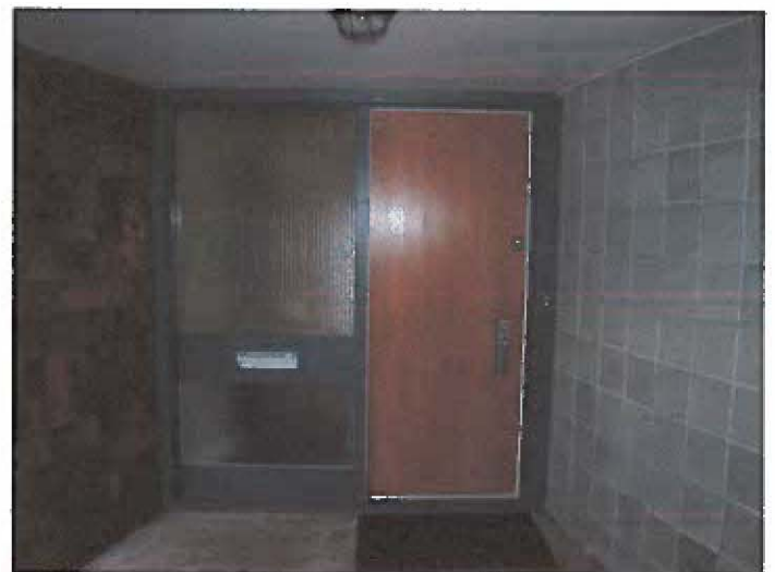
Original front door assembly with reeded sidelights
