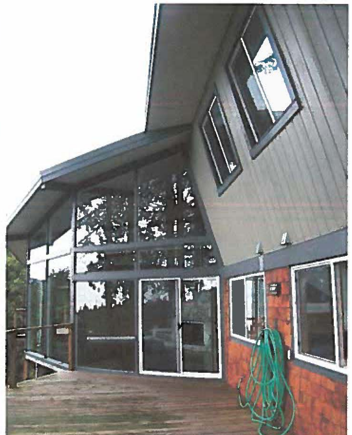
Angled upper wall with original wood siding, lower level with new cedar shingles
