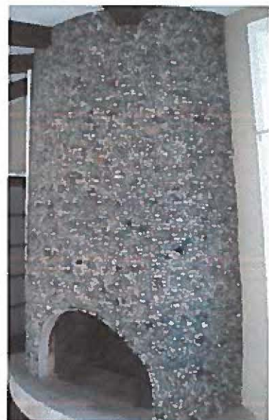
Original concrete block fireplace. Decorative pebbles are a later intervention.
