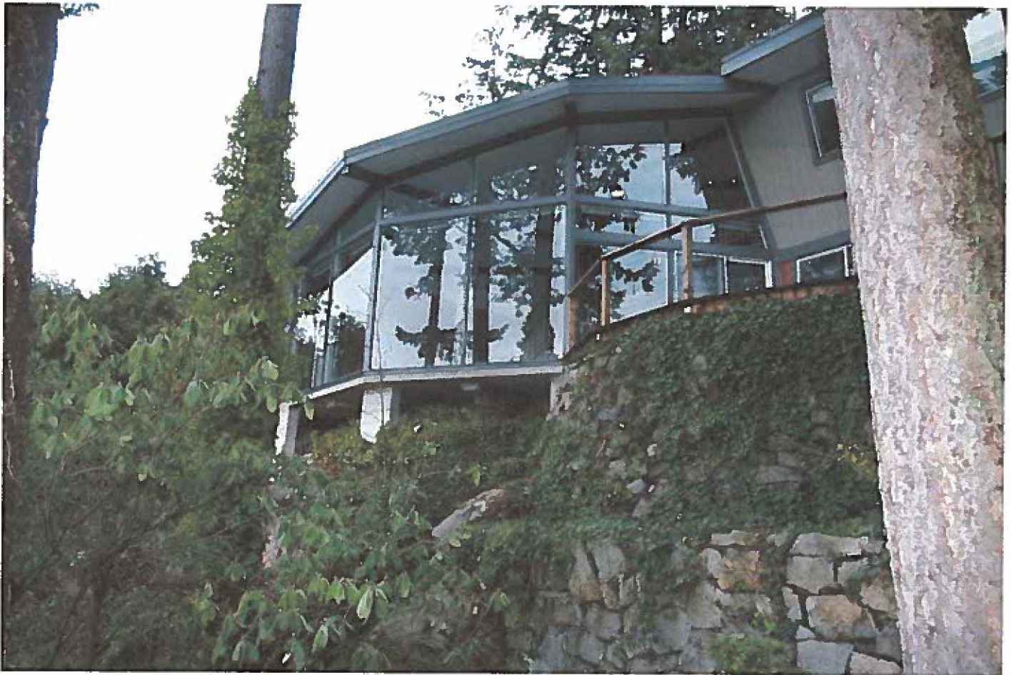
South view of the elevated Sykes Residence
