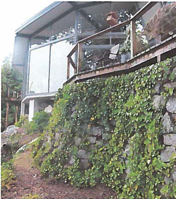
Granite retaining wall covered with ivy
