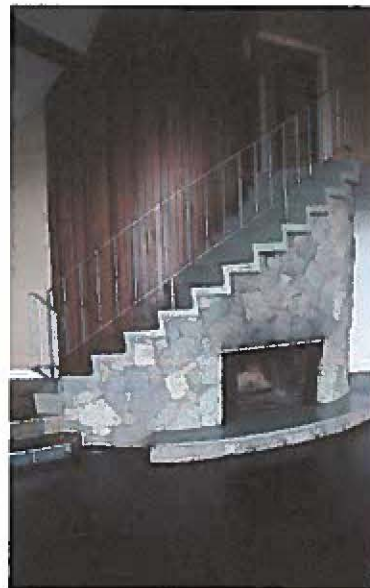
Concrete stair above granite-faced fireplace
