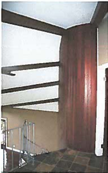
Original wood clad wall and beams
