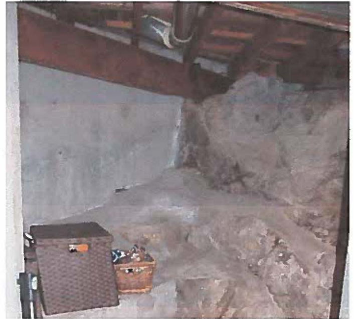
Concrete foundation wall built into bedrock
