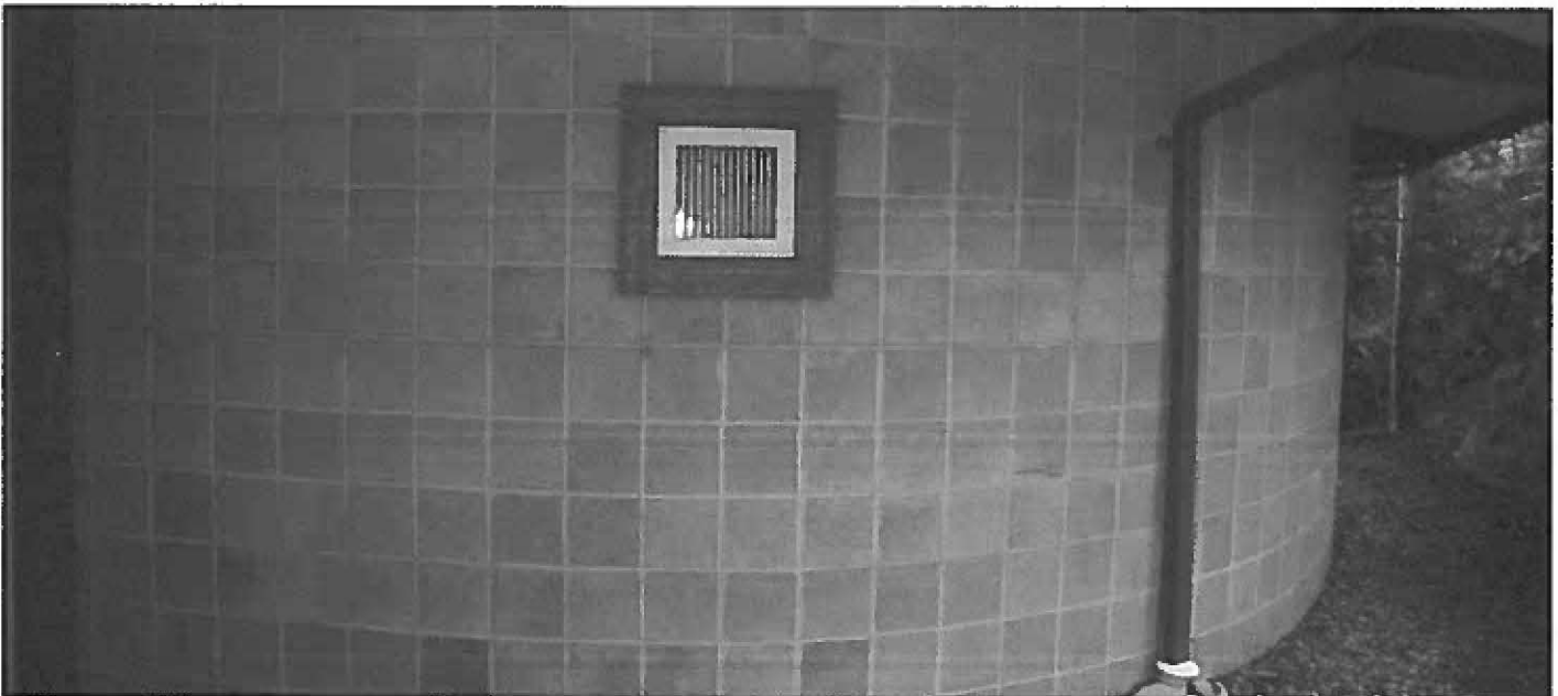
Original 'Denstone' block wall
