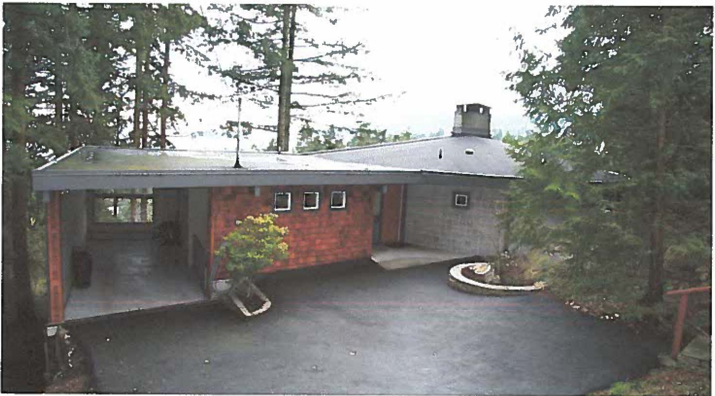
Flat roof above carport and office
