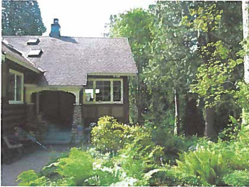
Left: Side-entry porch at west elevation return, showing chimney stack above the roof ridge, and the landscaping on the foreground.
