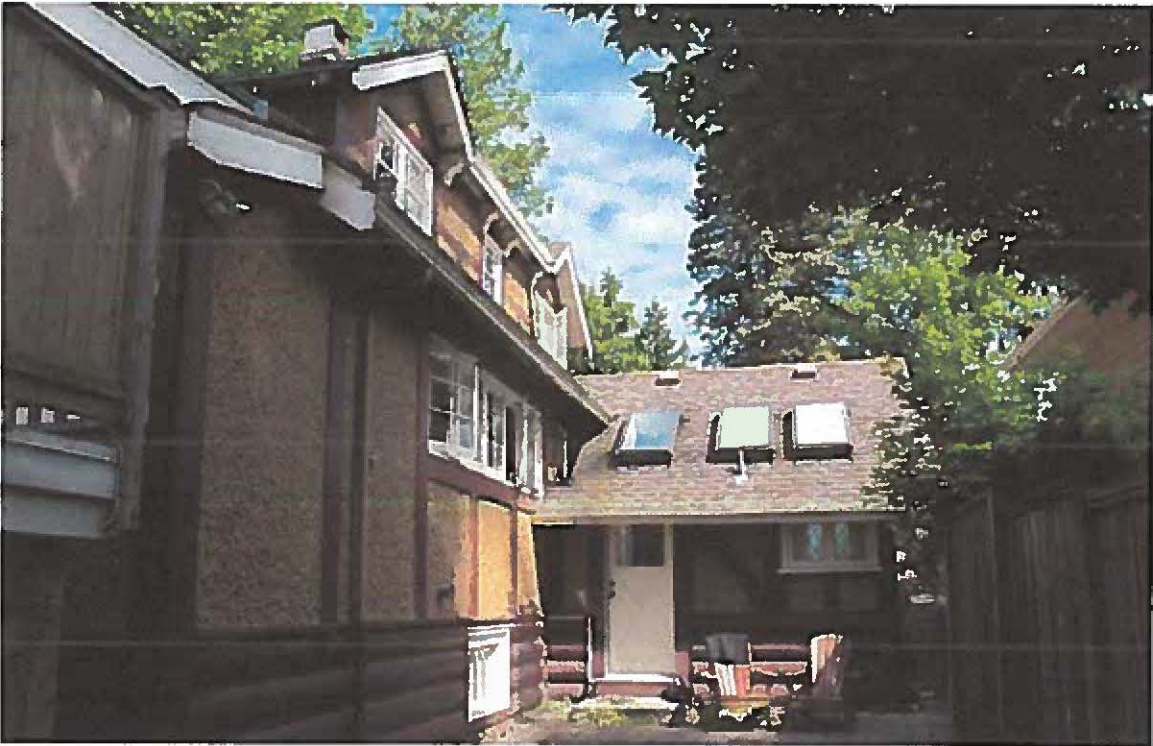
Partial east elevation and later side-gabled extension.
