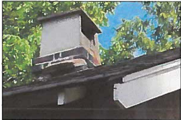
Existing rectangular chimneys: chimney with metal flashing above roof ridge of side-gable (top); and brick chimney with metal chimney cap above roof line to the south.
