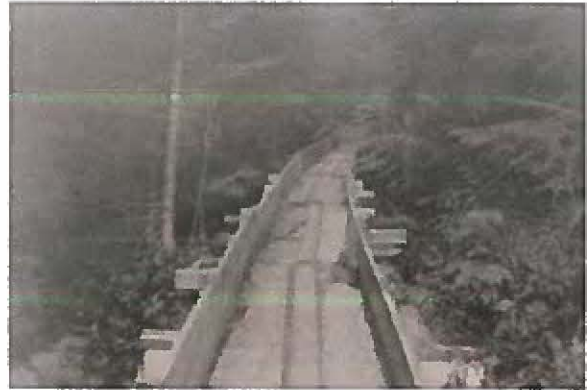
Example of a wooden box flume used to transport wood in West Vancouver, WVML 1634
