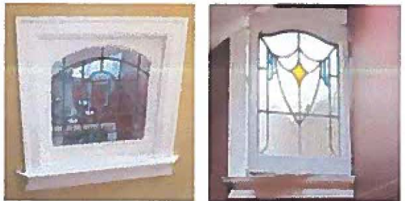
Photos showing existing interior multi-pane stained and leaded glass windows that were formerly exterior windows.
