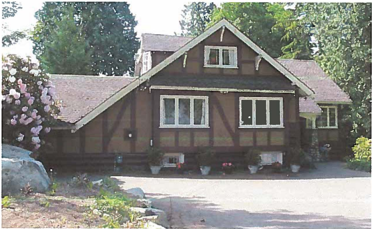
Front facade (North Elevation) of the Sutherland House, as seen from Inglewood Avenue.
