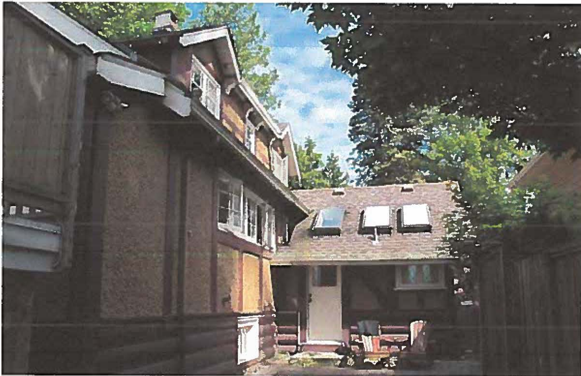
Partial east elevation and later side-gabled extension.
