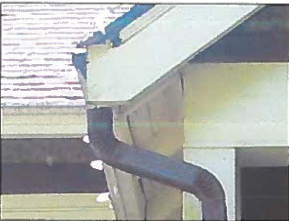
Cross-gabled roof structure of the Sutherland House (top); exposed roof rafters and nailing boards (middle); and typical condition of roof drainage (bottom)
