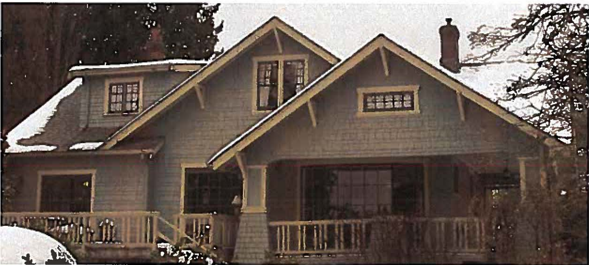
Photos showing original windows of the Rush House.
