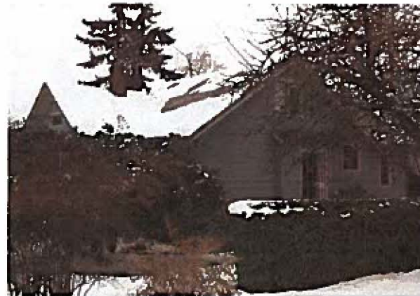
REAR elevation of the Rush House, at corner of 12th Street and Jefferson Avenue.
