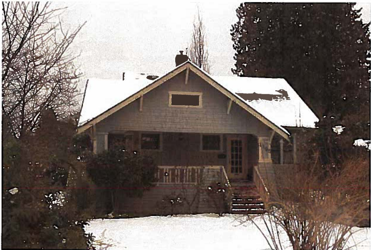
Historic front facade of the Rush House along 12th Street.
