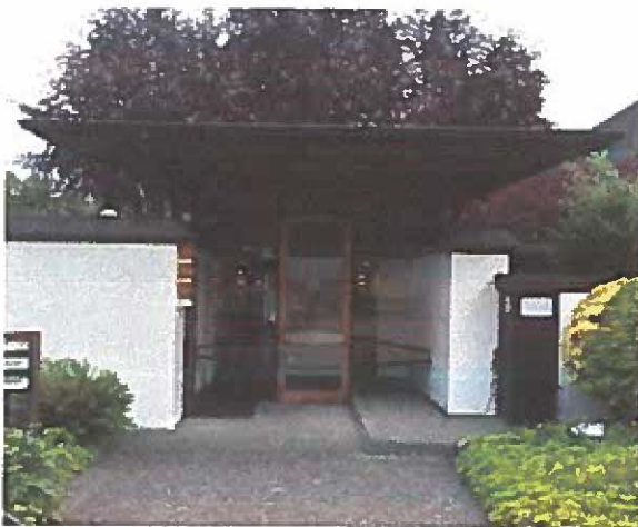
THE FRONT ENTRANCE
