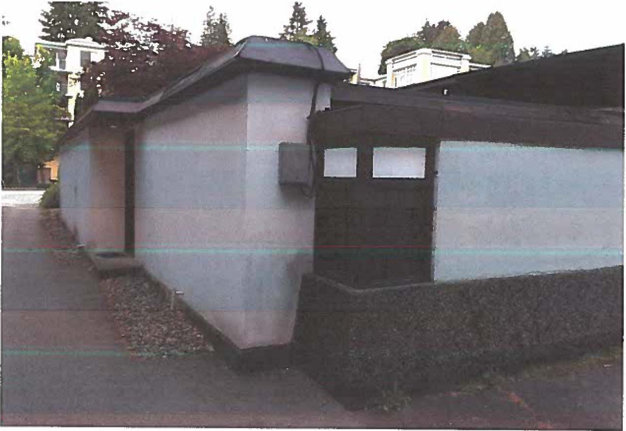
REAR OF THE BUILDING ABOVE: LOOKING NORTH BELOW: LOOKING ACROSS THE REAR NOTE THE CONCRETE SILL UNDER THE WEST WALL
