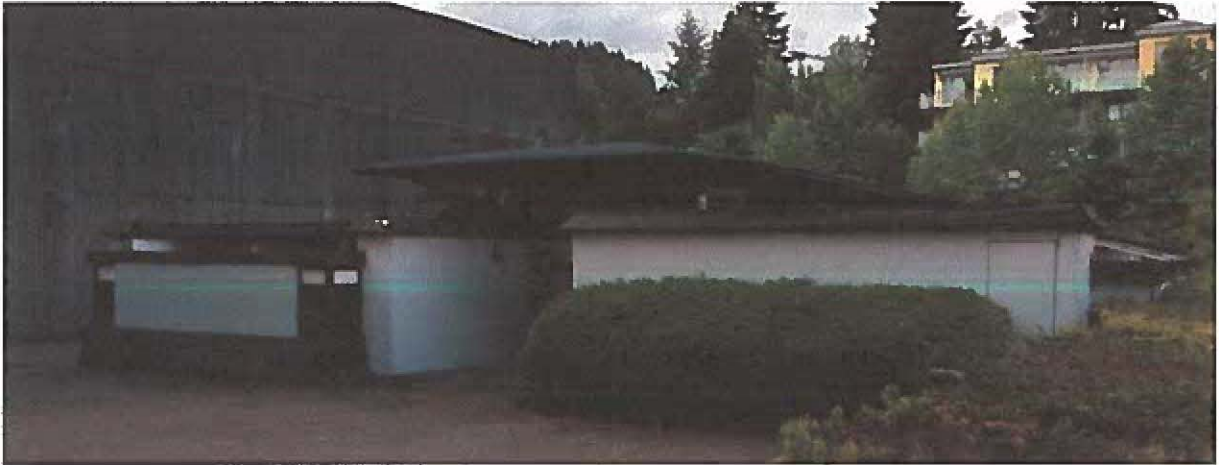
REAR OF THE BUILDING
