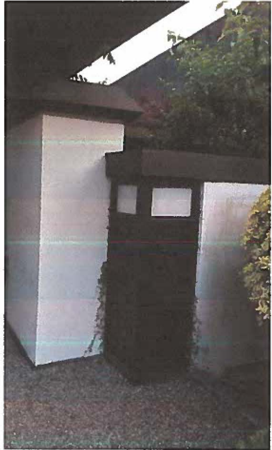
WOOD AND PLEXIGLASS PIERS WHICH ILLUMINATE THE BUILDINGS CORNERS IN THE EVENING
