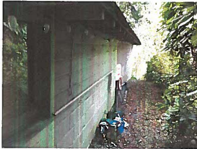
VIEW LOOKING NORTH ALONG EAST ELEVATION
