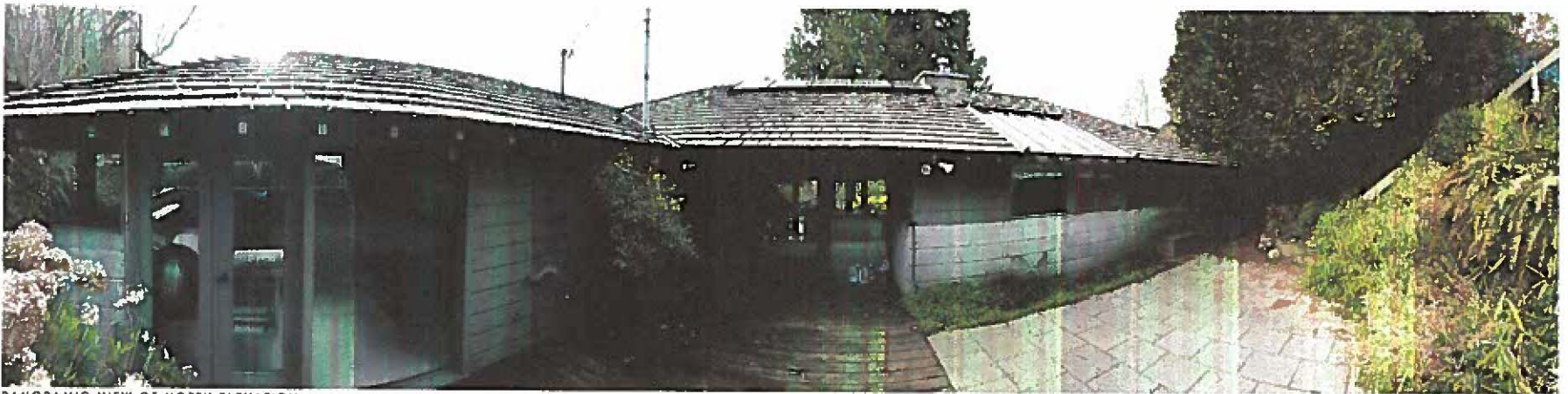
PANORAMIC VIEW OF NORTH ELEVATION
