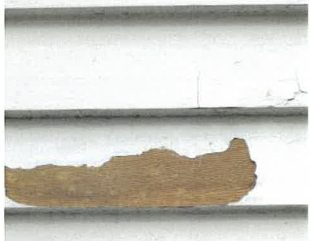
Figure 62: Natural look of siding beneath the white paint
