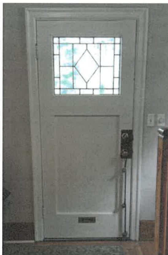
Figure 55: Front door interior
