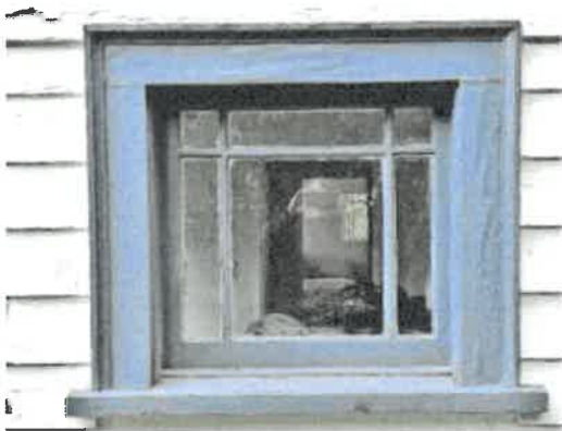
Figure 48: Basement window (WE-5)
