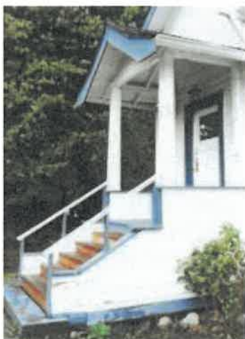
Figure 30: Front porch and stairs
