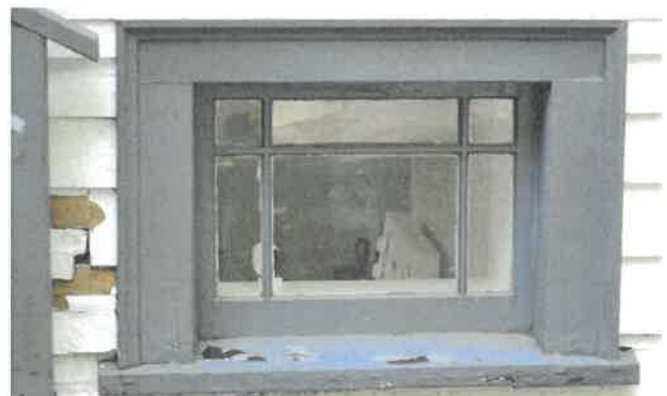
Figure 49: Basement window (WN-5)
