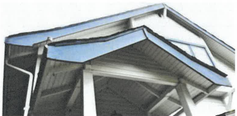
Figure 31: Front porch barge board and overhang
