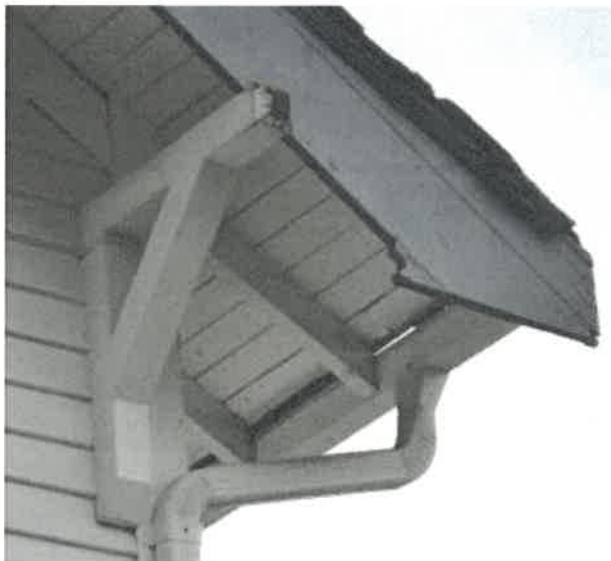
Figure 19: Open soffit with exposed rafters, bracket, and barge board
