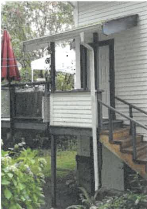
Figure 34: Back porch with roof, landing, and doors
