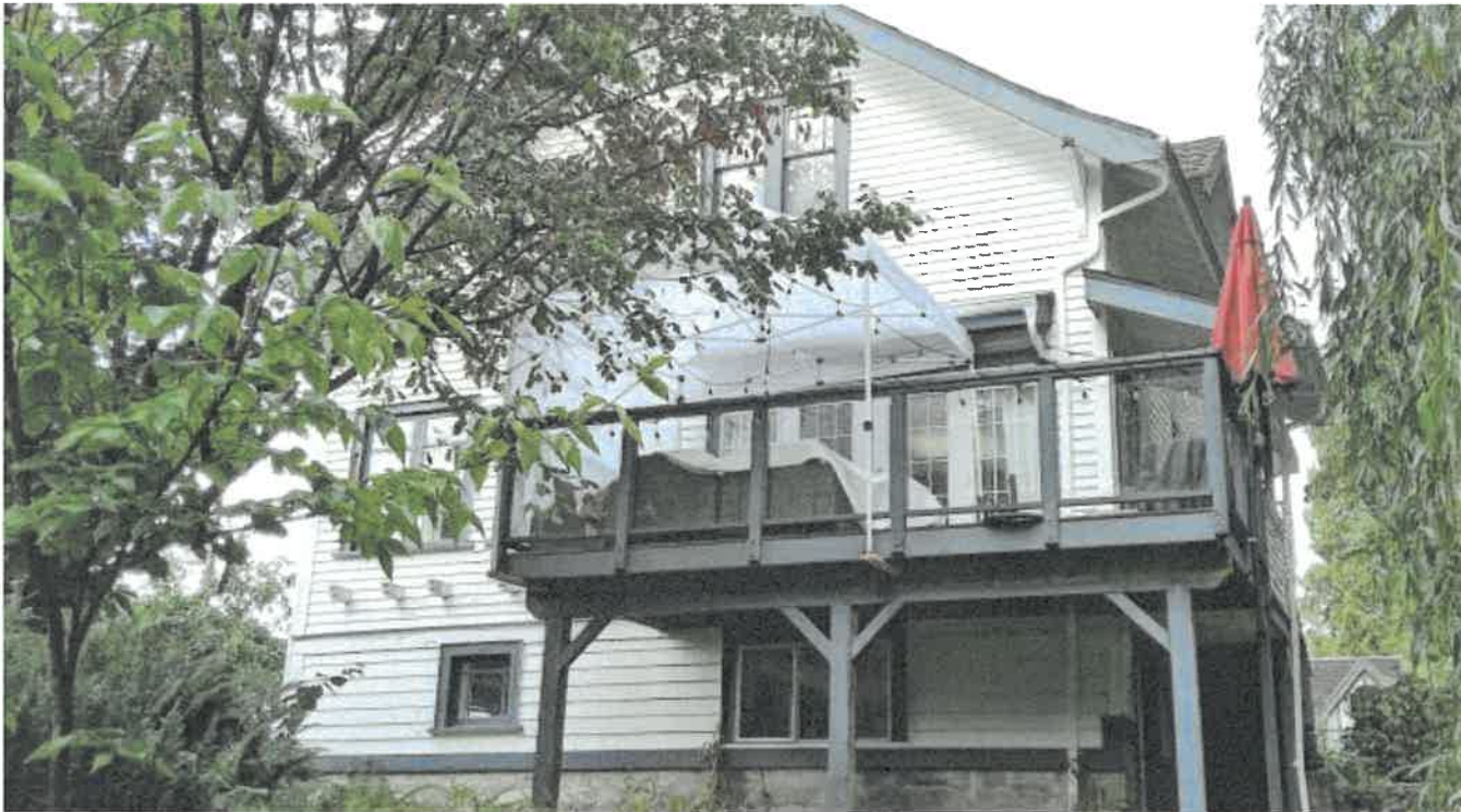
Figure 9: East elevation with deck
