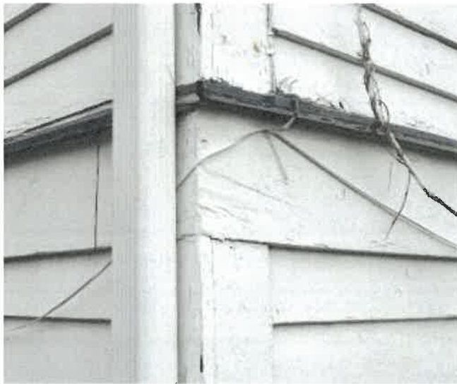
Figure 24: Lap siding, Water Table, Belt and Corner boards,
