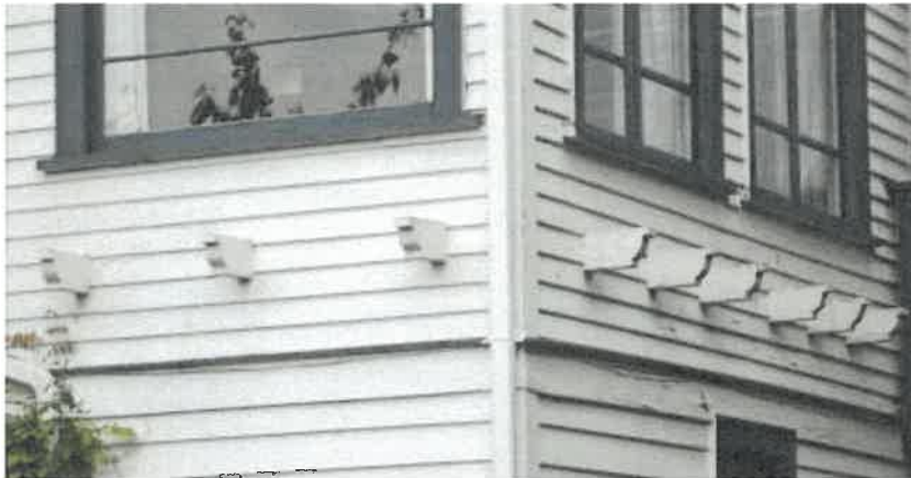
Figure 28: South and east elevation flower box studs
