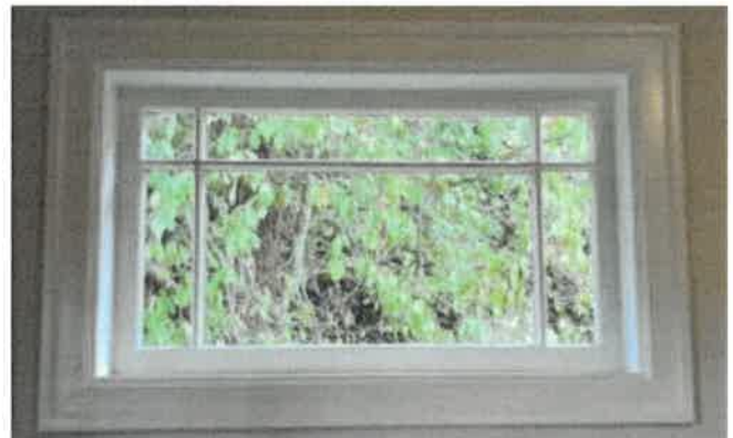
Figure 47: Interior of stairs landing window (WN-2)
