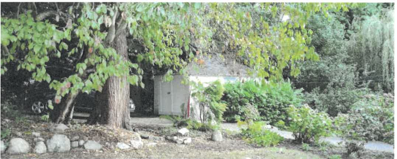
Figure 17: Garage on the north side of the property
