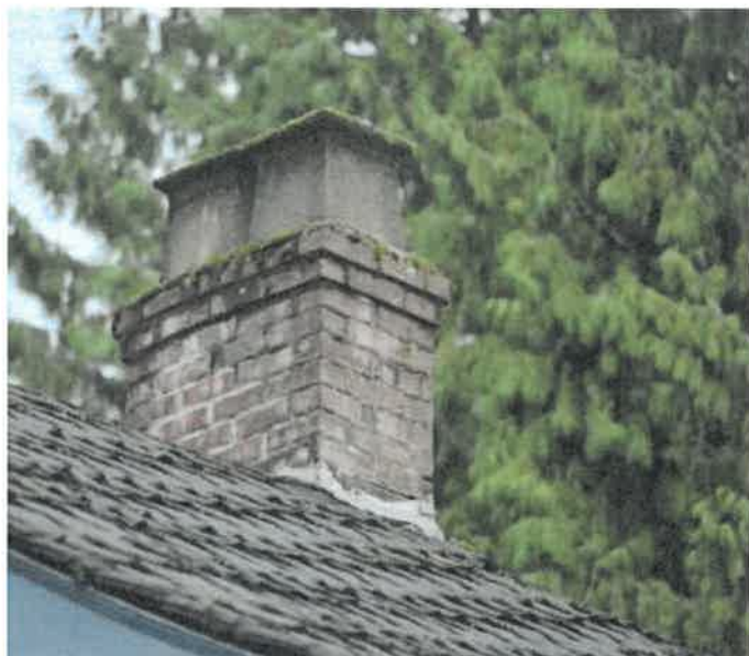
Figure 58: Internal chimney shaft above roof
