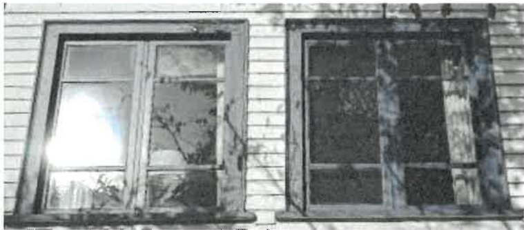
Figure 42: Two pairs of multi pane fixed and casement windows- (WE-1 & WE-2)
