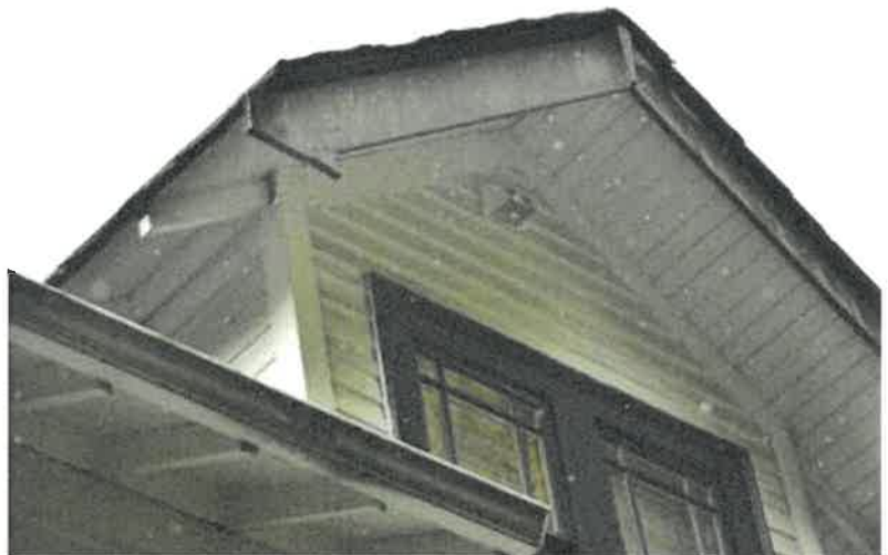
Figure 23: Front of typical dormer with bargeboard, exposed rafter and open soffit
