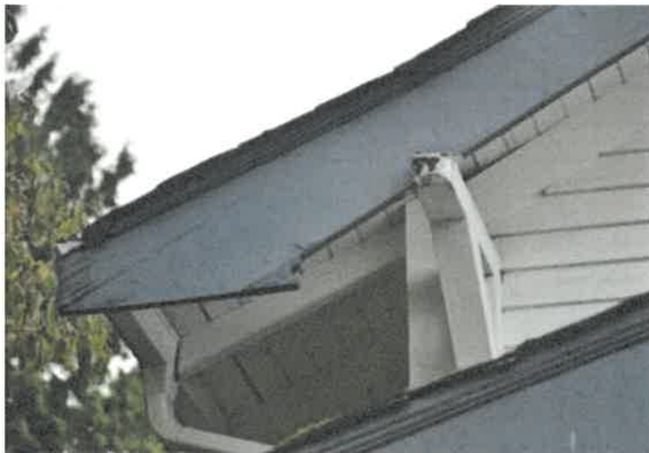
Figure 26: Headboard above siding
