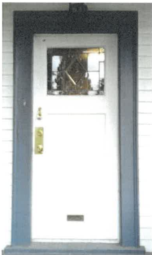
Figure 54: Front door exterior
