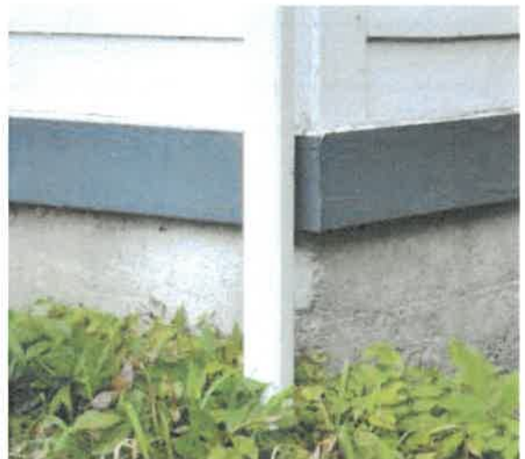
Figure 27: Base plate below siding
