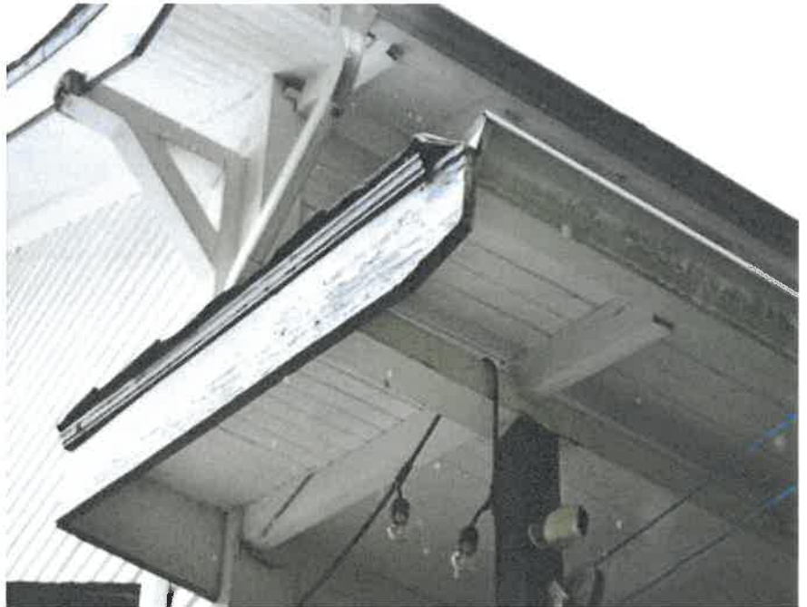
Figure 35: Back porch roof structure with barge board and exposed rafters
