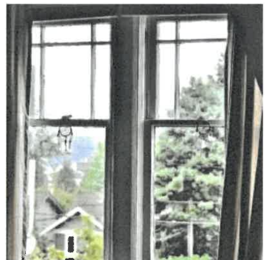
Figure 41: Interior side of pair of bedroom windows (WS-4)
