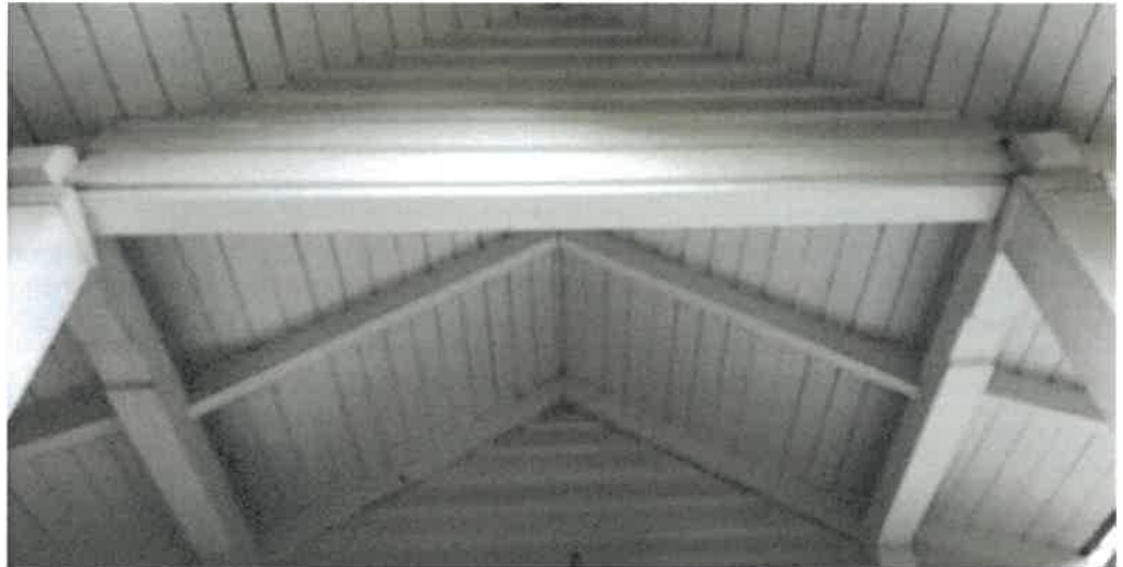
Figure 33: Front porch roof structure with clad tympanum in the foreground
