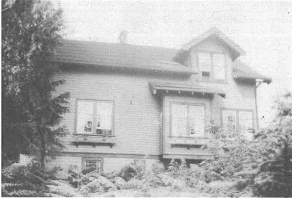
Figure 84: South Elevation of Clegg House, circa 1933
