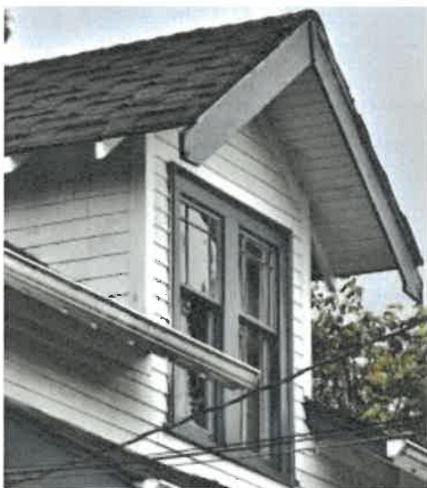
Figure 22: Shingle dormer cheek at south elevation
