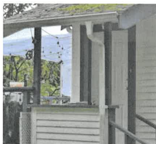
Figure 57: Back porch door
