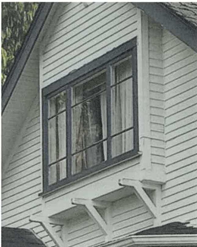
Figure 52: Box window with knee-brackets (WW-2)
