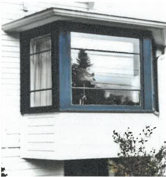
Figure 50: Multi pane bay window (WW-1)
