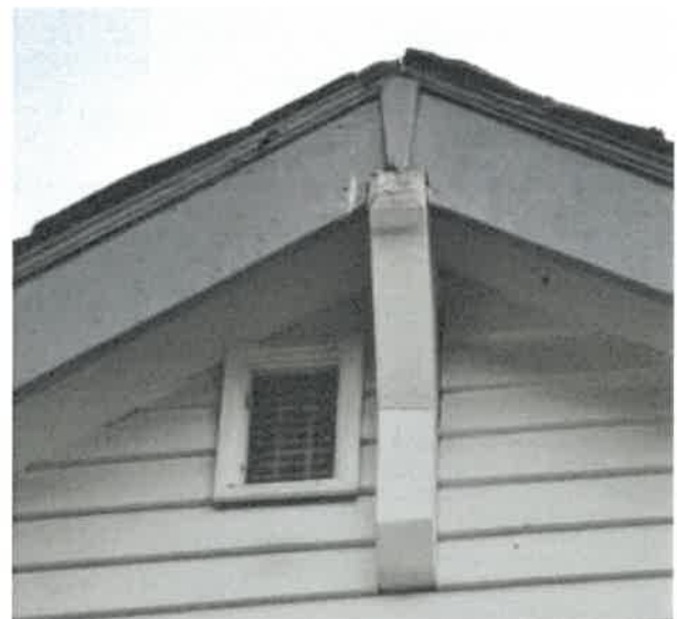
Figure 20: Knee-bracket at gable end's, moulding and key with attic vent
