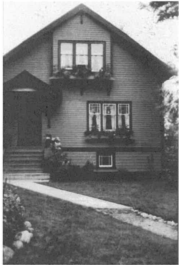
Figure 70: Front elevation with original porch brackets flower boxes and double hung windows photo from the Clegg family
