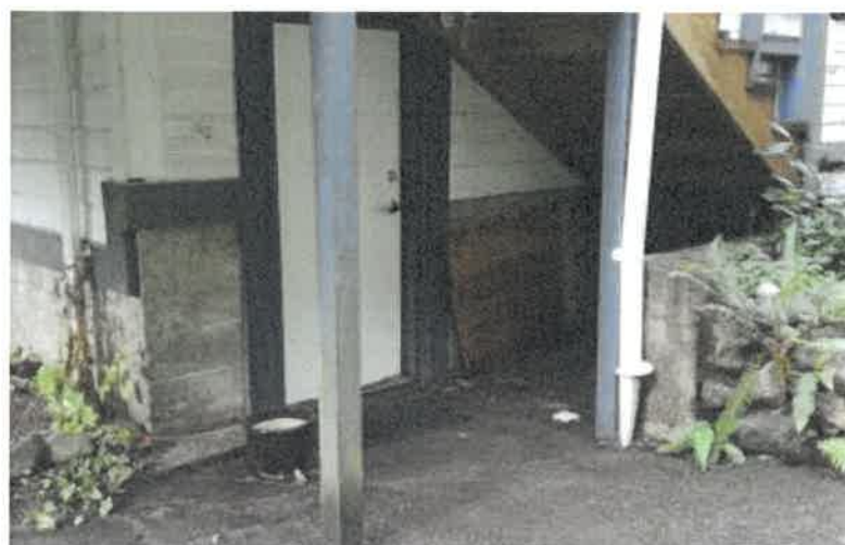
Figure 56: Basement door under back porch landing
