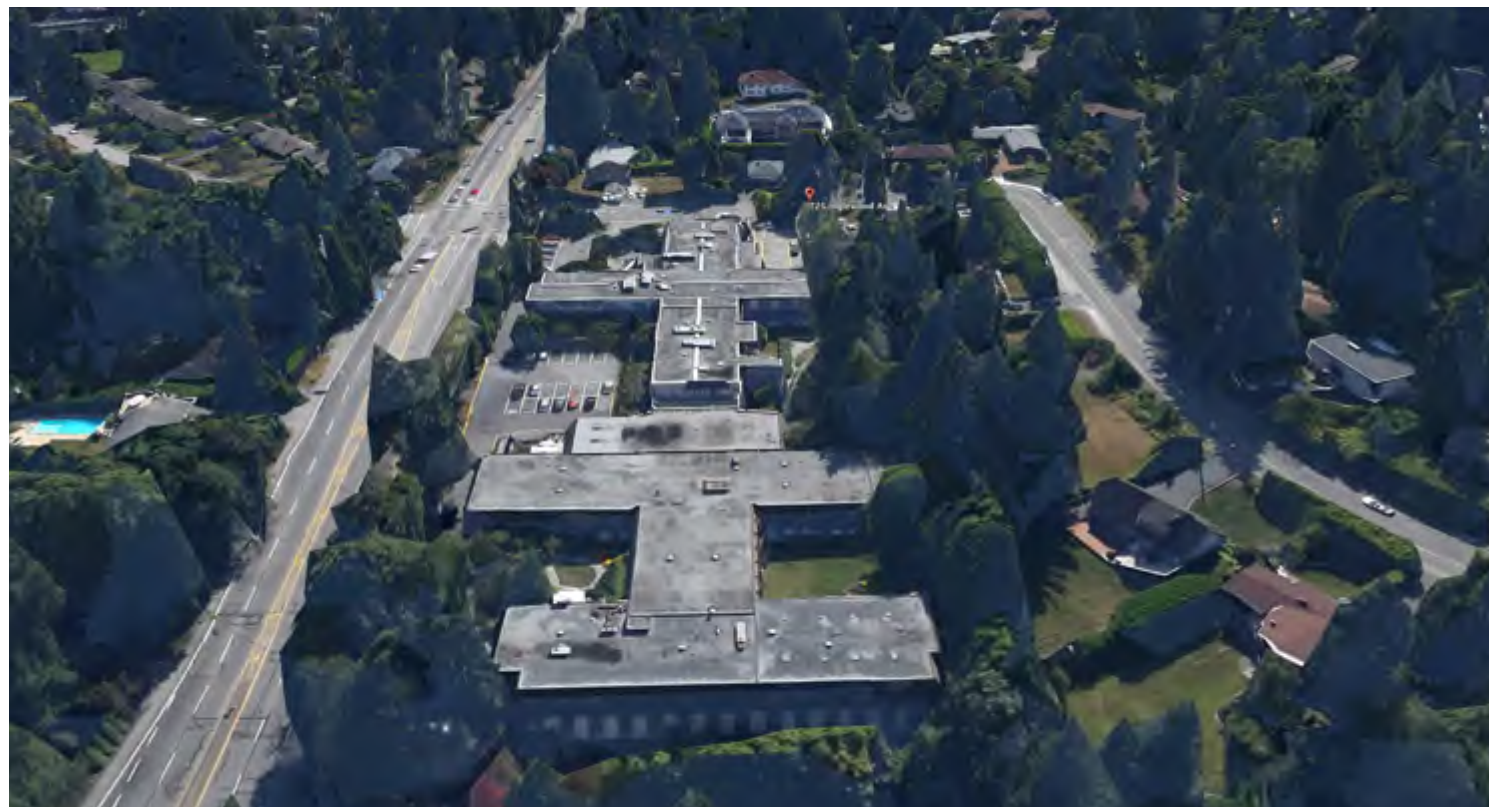
View from North
