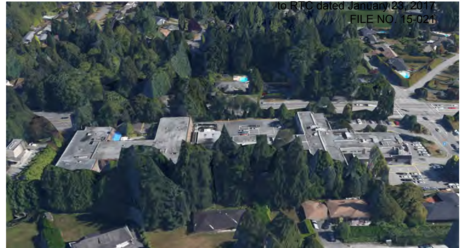
View from West
