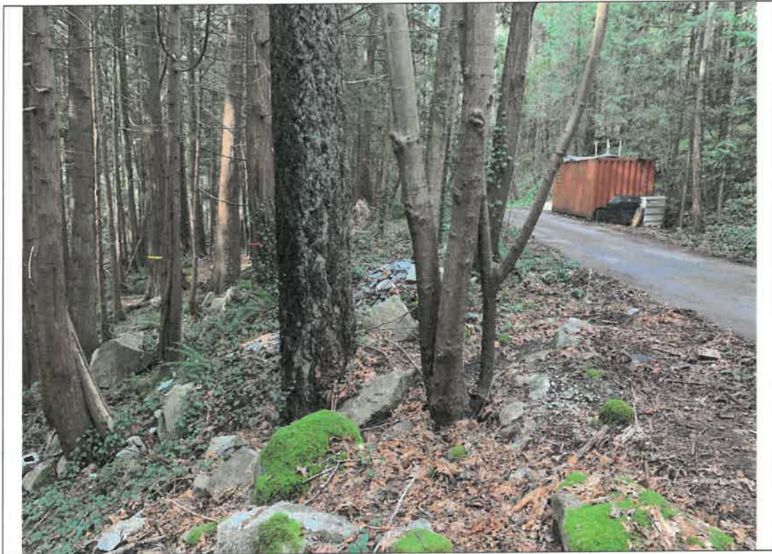
Slope beneath the driveway off Westport Road, looking northwest
