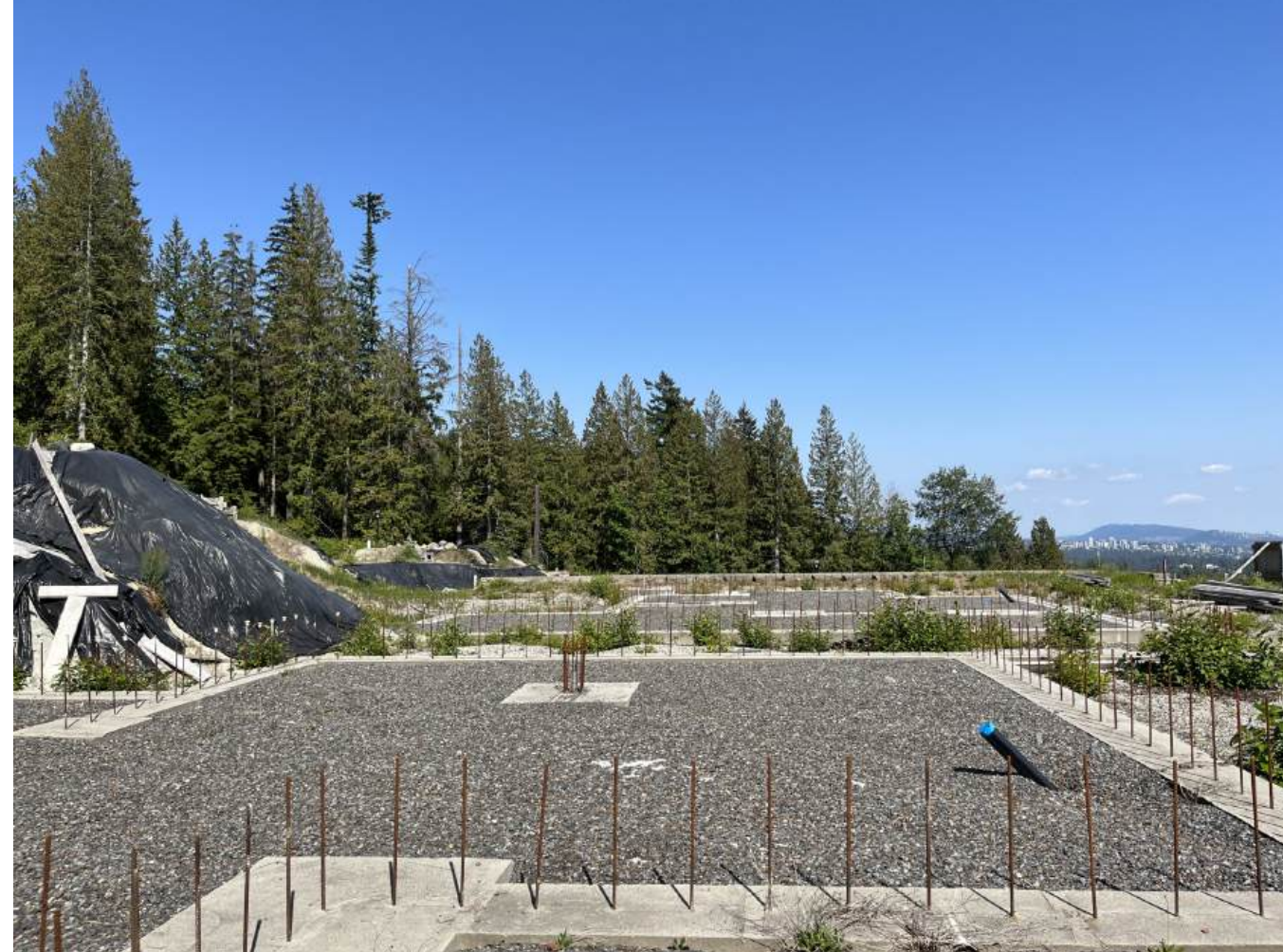
4 VIEW EAST FROM LOT 4
