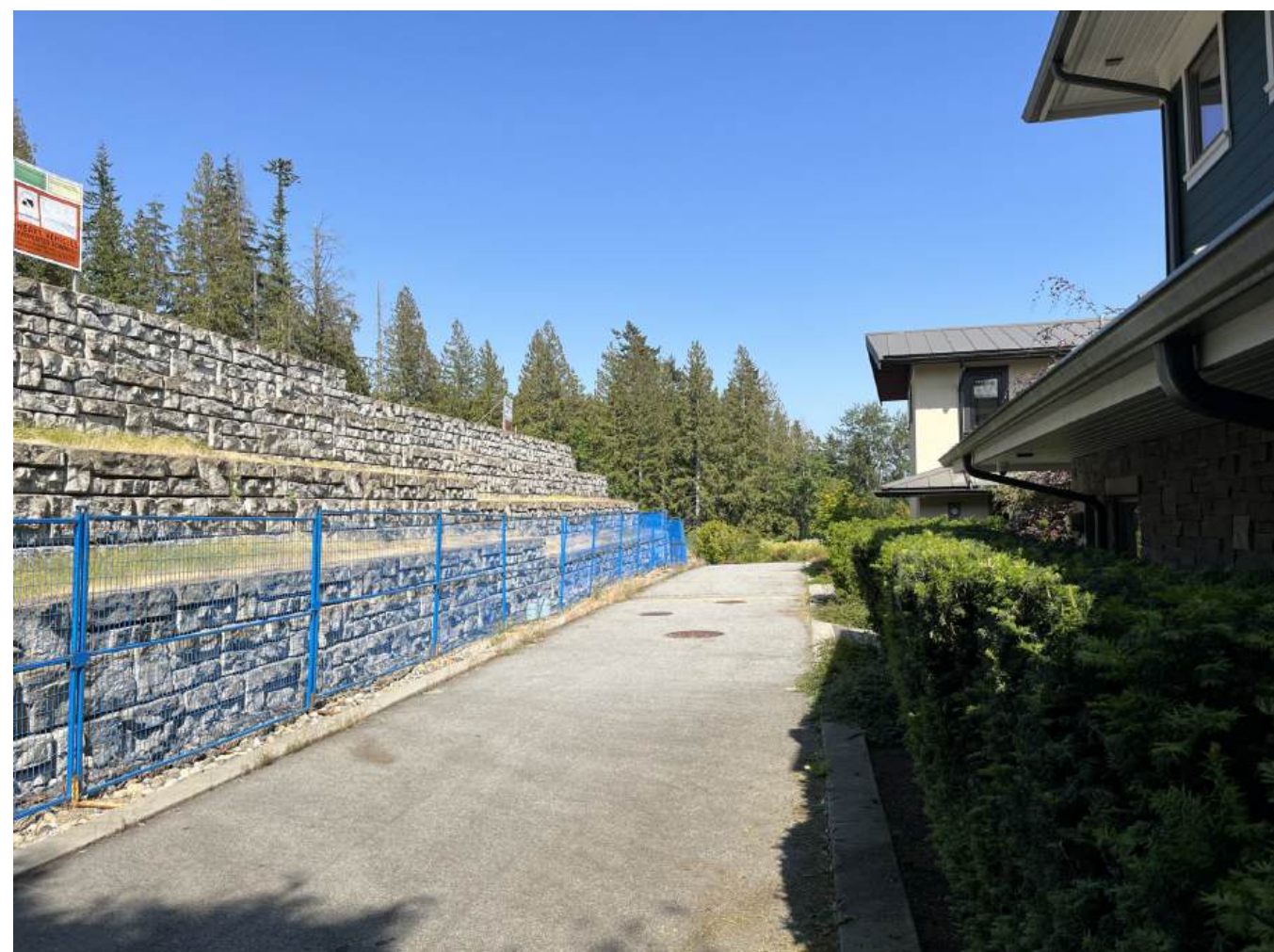
5 VIEW OF NEW ROAD OFF OF UNION COURT
