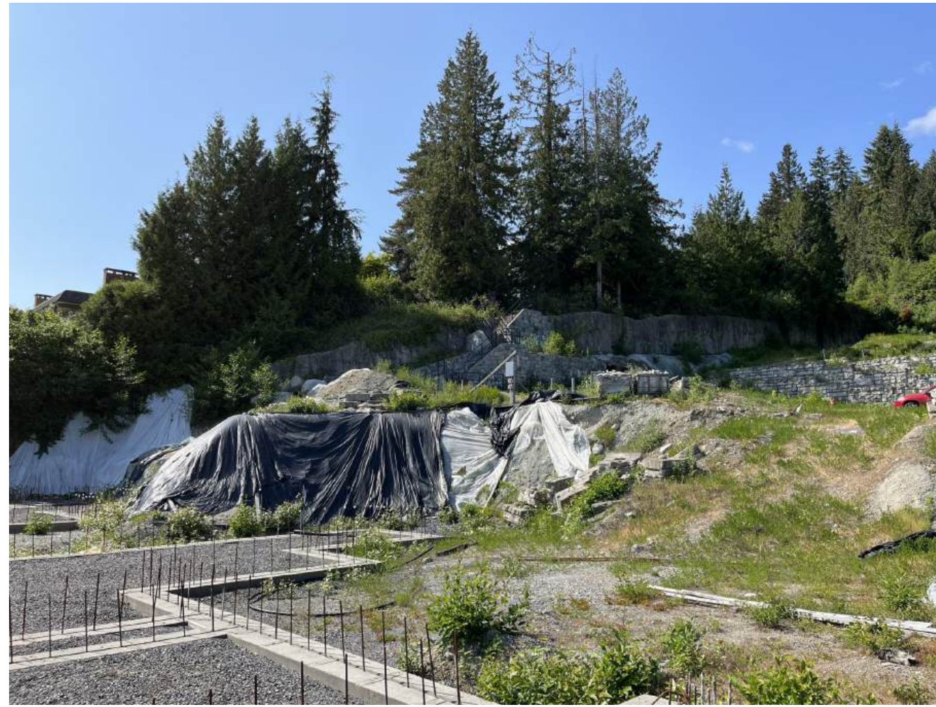
2 VIEW OF WEST PROPERTY LINE AND STAIR ACCESS TO TRAIL
