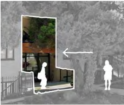
4.5.3 Recess entryways for weather protection
